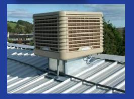
**External – Roof Mounted -** The building is ventilated using the evaporative cooler to provide a constant source of cooled air. The system is balanced using extract ventilation.
