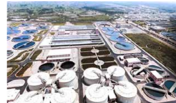
Jabl Asfar Wastewater Treatment Plant (Egypt) Optimisation: supply of the activation Technology: Delta Hybrid 9 x GM150S, 4 x GM30L Wastewater: 2 million m 3 /day Size: 14,000,000 equivalent population Savings: 25%
