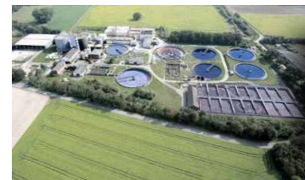
Rheda-Wiedenbrück Wastewater Treatment Plant Optimisation: activation Technology: Aerzen Turbo 1 x AT150 0.8S, Delta Hybrid 1 x D62S, Delta Blower 2 x GM80L, AERsmart Wastewater: 3000 m 3 /h Size: 20.000 population equivalent, 326,000 population equivalent Industry Savings: €40,000 per year
