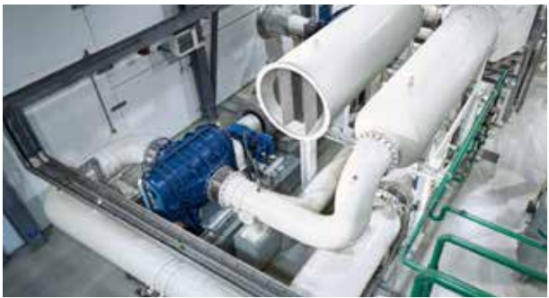
Plant for the production of oxygen
