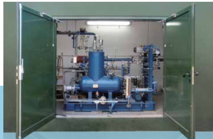
AERZEN VMX 110 compressor for the compression of biomethane
